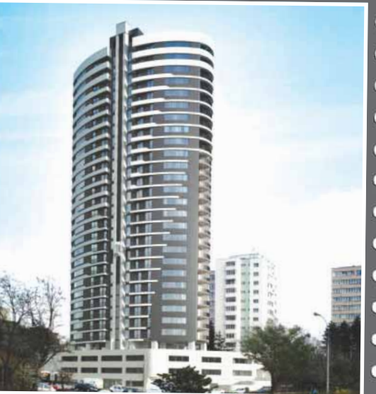
West City Tower
